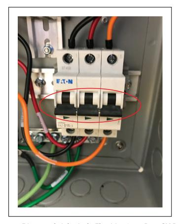
Figure 2-24. Disconnect Switches in the Electrician Access Box - ON Position
