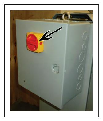
Figure 2-15. Main Disconnect Switch Placed in OFF Position
