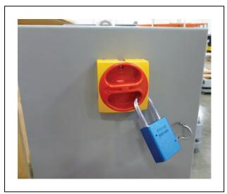
Figure 2-16. Main Disconnect Switch Locked
